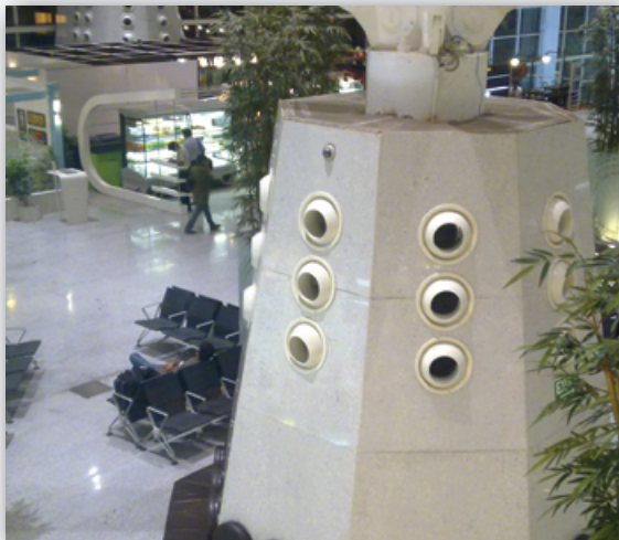
JET NOZZELS INSTALLED AT AN AIRPORT
